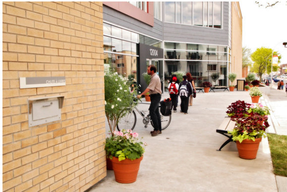
Cultural and Community House in North-Montreal. Photo: Caroline Durocher.
