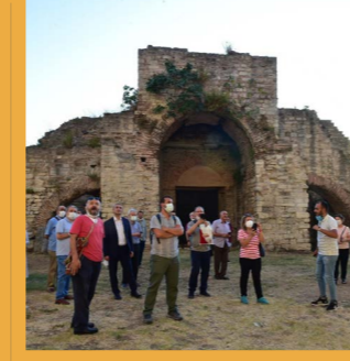
13. Fatih: Yedikule Fortress Restoration and Culture and Art Space Project
